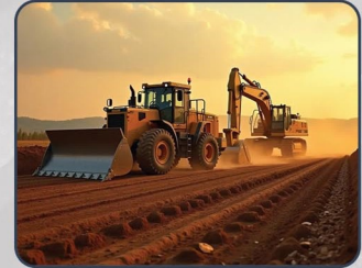
Road Construction Equipment
